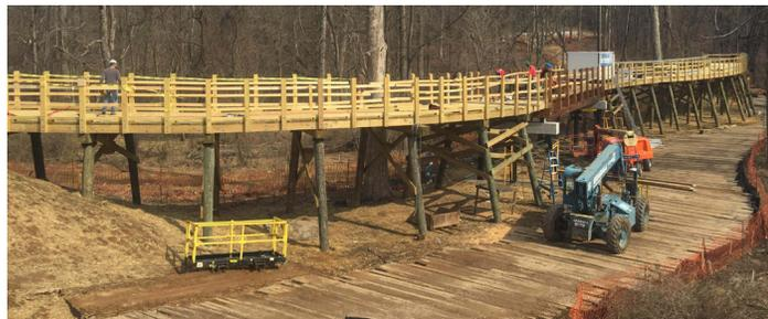
A temporary 20' wide x 680' long "corduroy road" was built to provide a foundation for the heavy equipment while building the Stevenson University pedestrian bridge.
