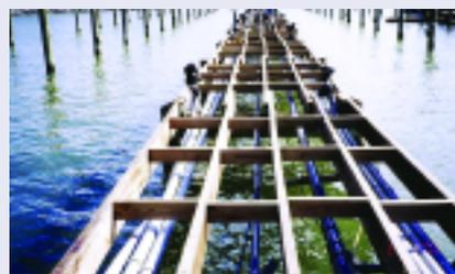
Figure 6. Typical framing configuration for fixed dock with utility runs.
