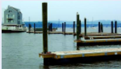
Figure 4. Typical finger arrangement on floating dock.
