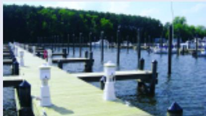
Figure 2. Fixed timber dock installation.
