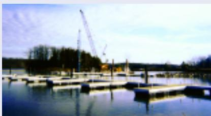
Figure 1. Pile-supported floating dock installation.
