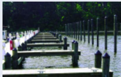
Figure 5. Typical finger arrangement on fixed timber dock.
