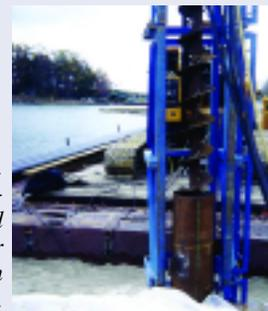
Figure 3. Crane-mounted augur for auguring in mooring piles.
